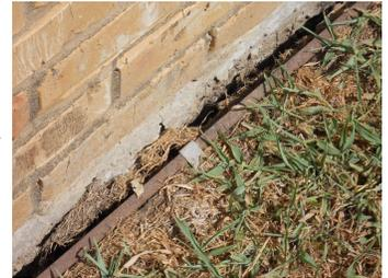
Crack that has opened up near foundation.
